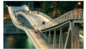
Passerelle Simone-de-Beauvoir, Paris 2006
